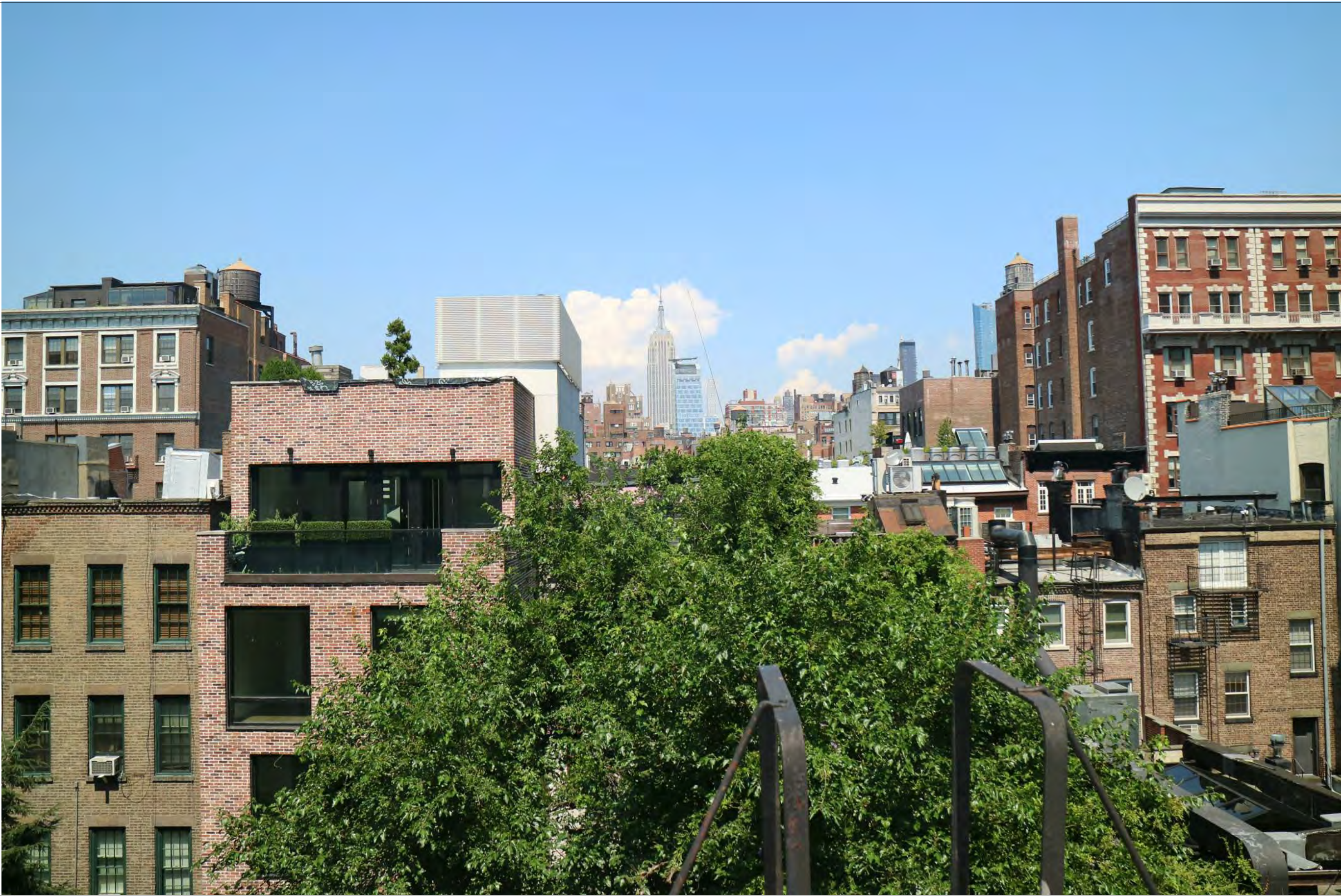
C3 PHOTOGRAPH - VIEW OF REAR FACADES
