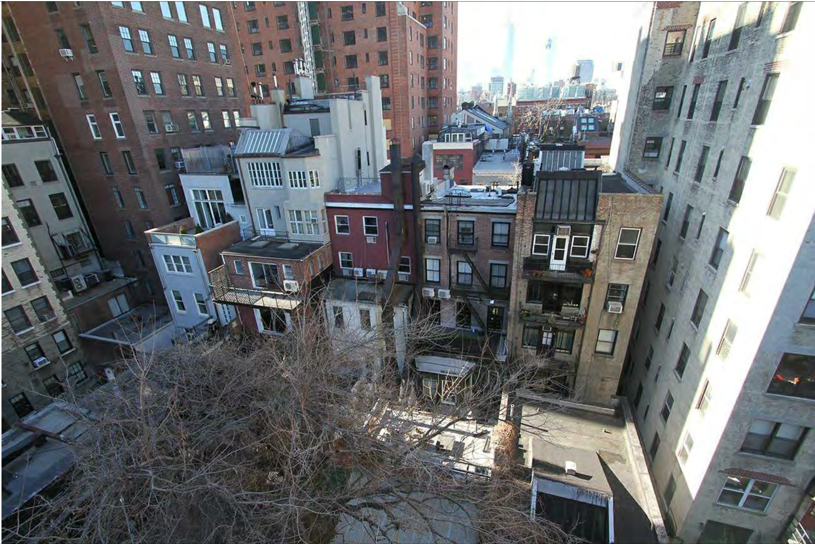
E3 PHOTOGRAPH - BIRD'S EYE VIEW OF REAR FACADES
